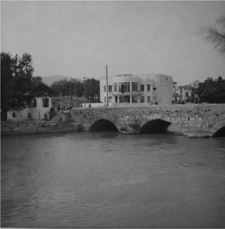
FIGURE 11.2 The Parliament building and the Roman bridge over the Orontes
